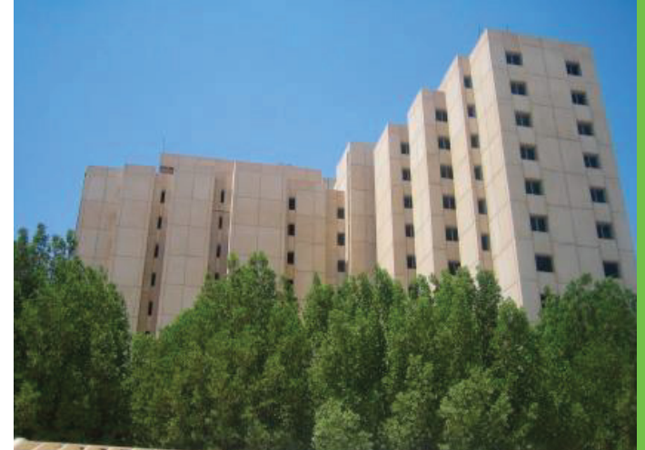
UNIV. TEACHERS ACCOMODATION - Shuwaikh
